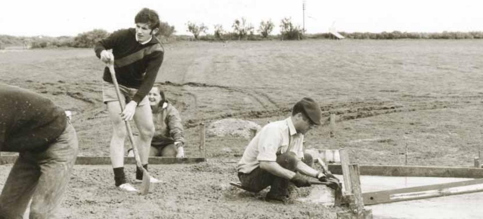
ABOVE *Laying the foundations and slab for the SASPC clubhouse at Lower Light in 1971 under the direction of Army engineer Mike Tonks (right).*
